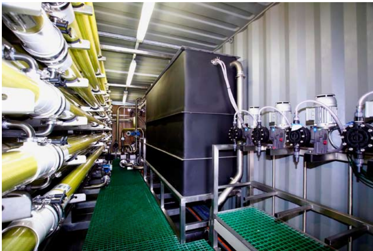
Containerised systems are used as mobile leachate systems for landfill sites.
